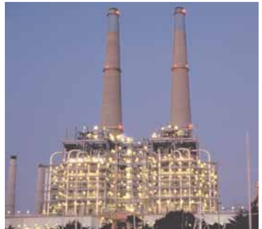
SIC works in power plants throughout the U.S.
