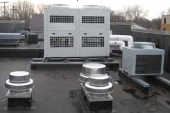
Air-cooled Chiller for the MRI
