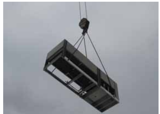
An industrial refrigeration project at Vicorp
